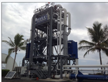
Figure 2-8 – Makai closed cycle 100kW test facility at NELHA. Right hand picture shows OTEC plus aquaculture-related facilities.
